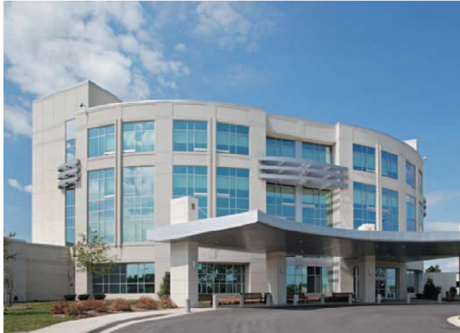
Figure 7: An example of a building with Solarban 80 windows
